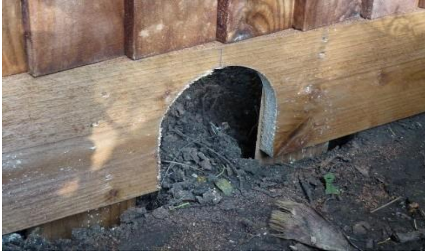
Hedgehog hole in fence – fences can also be installed with a gap at the bottom
